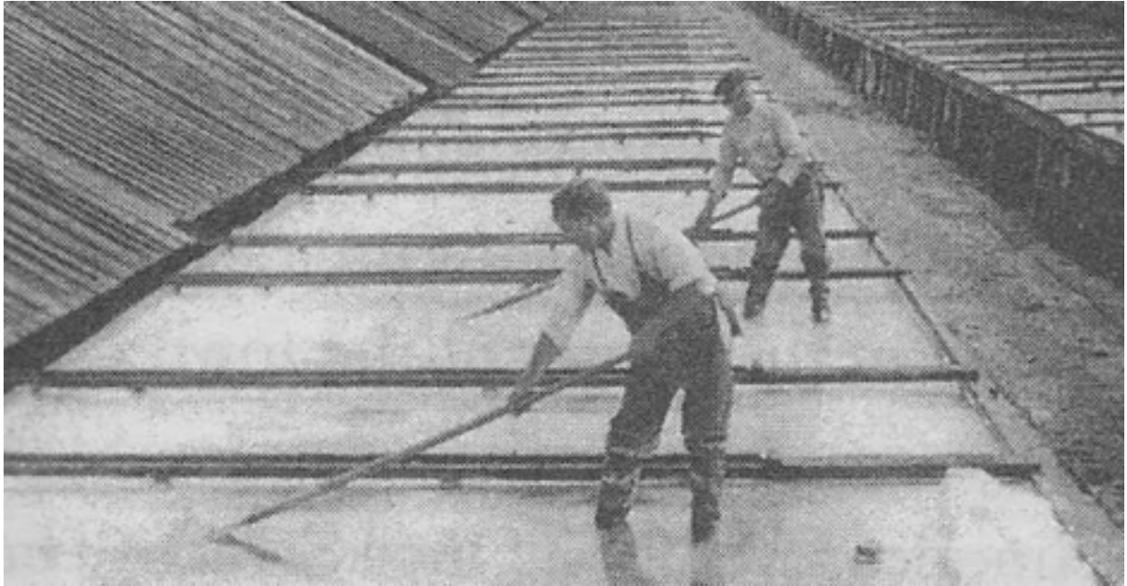
Onondaga saltworks showing salt being raked from solar evaporation vats of a design copied from the Cape Cod saltworks.
